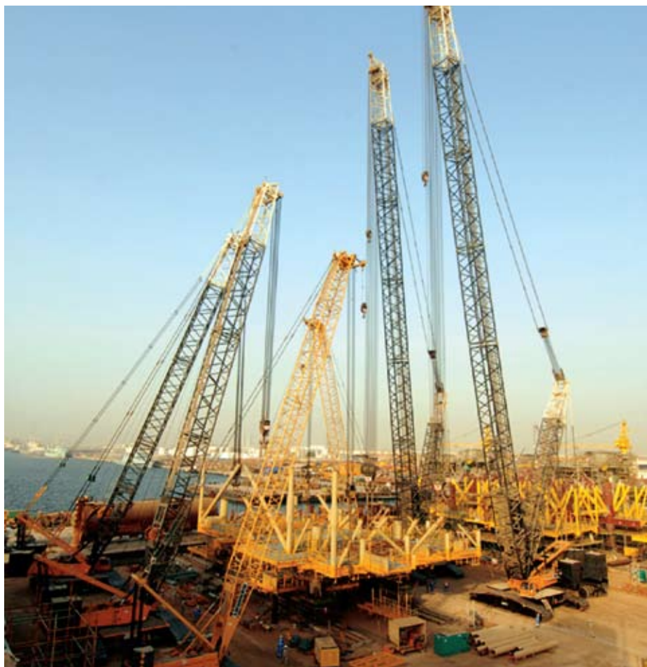
Pearl 1 and 2 topsides in Jebel Ali fabrication yard, Dubai
