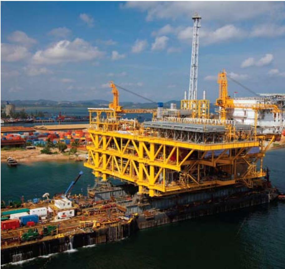
Su Tu Vang deck load-out was completed August 6-8 for transport to its final destination: Vietnam's Mekong Basin.
