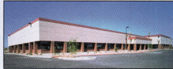
Plumwood Office Bldgs. 156,630 s.f.
